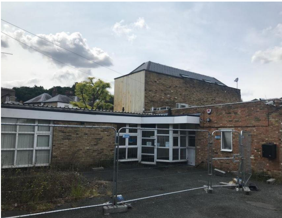
Photograph 2 internal site looking southwest towards The Studio.
