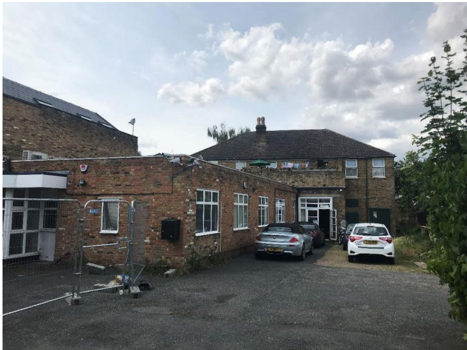
Photograph 4 internal site looking northwest towards existing maisonette.
