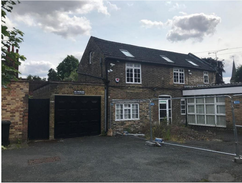
Photograph 3 internal site looking south east.
